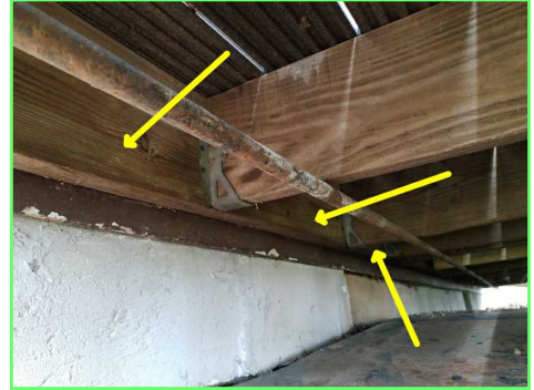
Not Properly Secured to House
