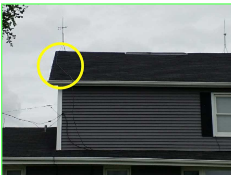
Missing Shingles
