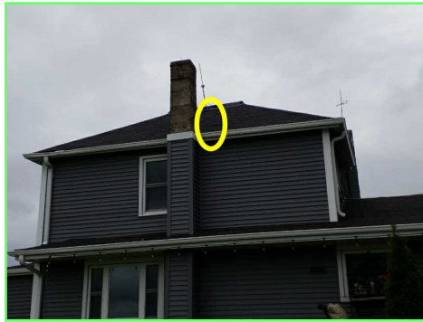
Missing Shingles
