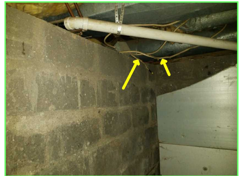
Abandoned Wiring
