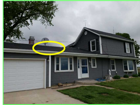
Missing Shingles
