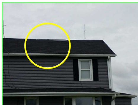
Missing Shingles
