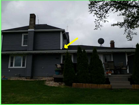
Discharges Onto Roof
