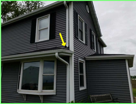
Discharges Onto Roof
