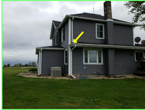
Discharges Onto Roof
