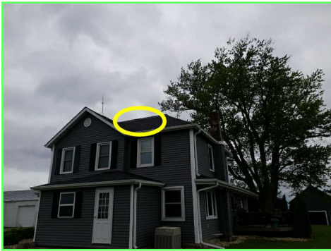
Missing Shingles
