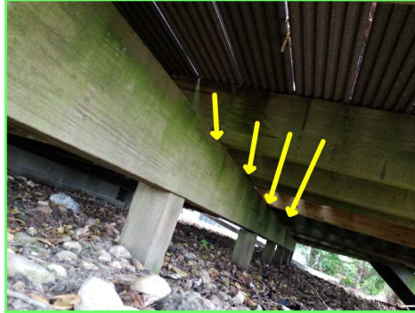
Floor Joists Not Secured Properly
