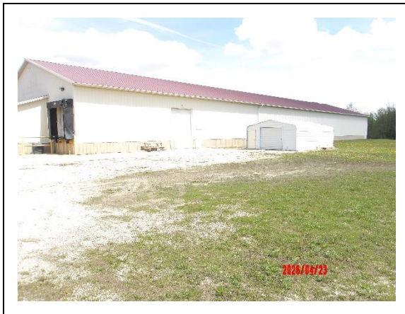
North - Side of Building
