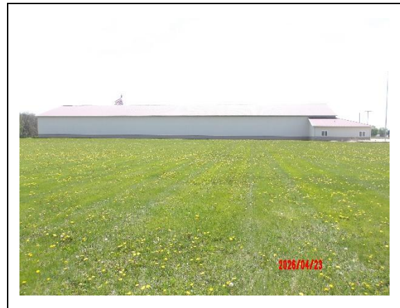
South - Side of Building
