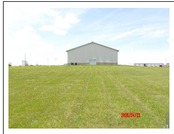
West - Back of Building
