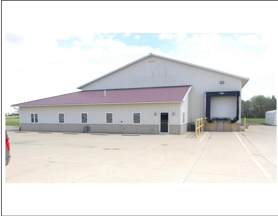
Vacant Warehouse 123 A Street Atown, IL 10010
